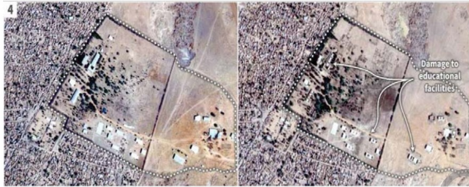
Satellite imagery showing damage to Zalingei University, School of Agriculture buildings east of Zalingei [12.93356,23.50195]. Obtained: 02 Mar 2023 (left), 11 Nov 2023 (right). Sources: Planet Labs PBC, Annotations by CIR.
