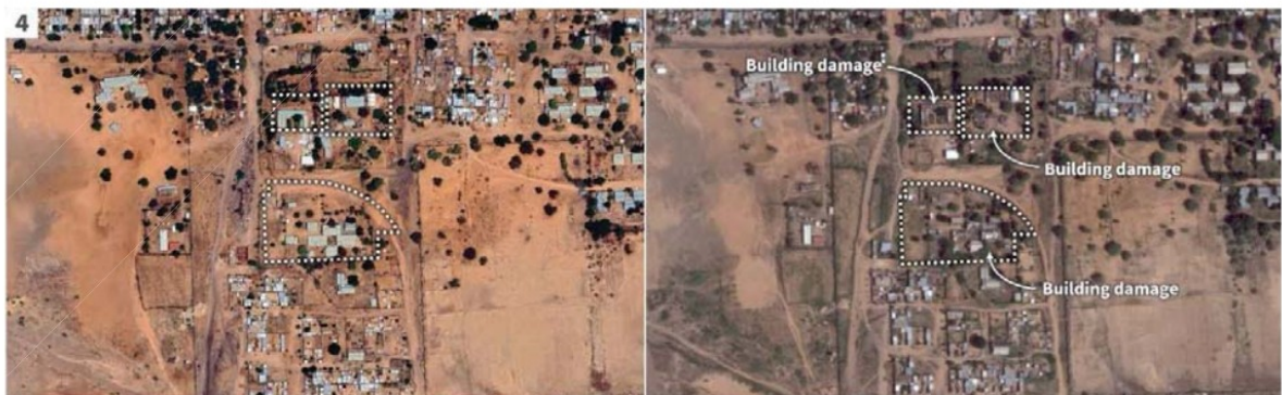
Satellite imagery showing damage to government and educational buildings in Karari East neighbourhood, Nyala, southeast from the SAF 16 Infantry Division. Obtained: 08 Apr 2023 (left), 24 October 2023 (right). Sources: Google Earth, Airbus DS, Planet Labs PBC, Annotations by the Centre for Information Resilience (CIR).
